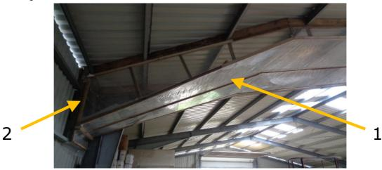
Fig. 2. Air collecting channel covered with polyethylene film: 1 – air collection channel; 2 – connection between the duct and air collection channel
